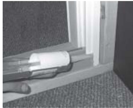
1) Place a bead of silicone at the operating jamb/sill corner along its perimeter.
