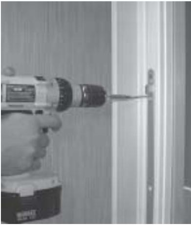
2) Once the keeper(s) are in position, replace the short factory installed screws with the (8) #10 x 3" screws from the installation screw pack. These long screws will insure that the keepers stay in place.
