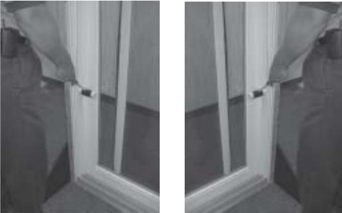
1) Take Jamb Covers and snap into the inner cavity on the jambs (A rubber mallet might be needed). Jamb covers will have one end with a notch in the middle (this end goes towards the sill) and one end with sides notched (this end goes into the head cavity).
