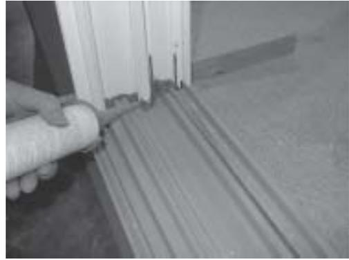
4) Place a continuous bead of silicone following the perimeter of the jamb from the top of the setting block, around the dividing wall and around the roller track tower until the entire perimeter is sealed.
