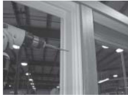
10) Use (5) #8 x 2" PH screws to fasten the astragal to the astragal panel end follow the groove and evenly space the screws.
