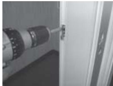
3) Screw in the keeper on the jamb (use marks that you made to align with lock) use two screws that were attached to the keeper with the screens.
