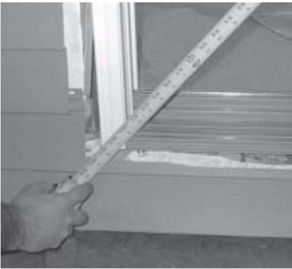
2) Center the door frame in the rough opening between its framing. This allows the frame to be squared and shimmed and also allows vinyl expansion and contraction with the seasons.
