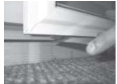
1) Insert the lock screen into the screen channel on the active side of the door (on the right from the outside) Insert the screen into the screen channel top end of the screen into the head first. Use a putty knife to push up the bottom rollers when inserting the bottom of the screen into the door.
