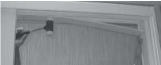
1) Take Head Cover and snap it into the outer cavity on the head (A rubber mallet might be needed). Head Cover will have two 90° ends.
