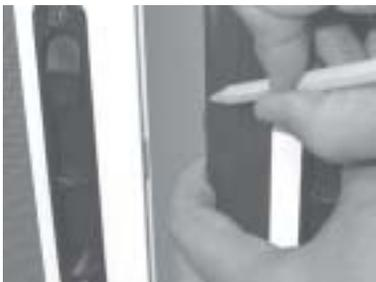
5) Align up the keeper to the lock and mark the keeper screen for keeper location.
