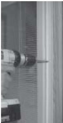
3) With the exterior of the panel facing you, locate a vertical groove next to the interior weather strip on the interlock. Use (5) #8 x 1" PH self drilling screws to fasten through the interlock into the face of the panel. Evenly space the screws down the full length of the interlock.
