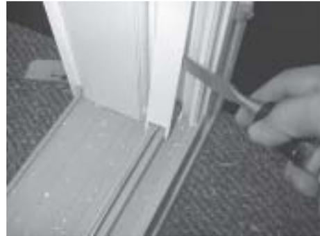
5) Remove Keeper and Infill cover from operating jamb by removing the two short screws from the keeper. Keep them together because you will be placing this back on later.
