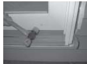
6) When the panel is completely engaged in the jamb pocket, check alignment of the interlocks for a good seal.
