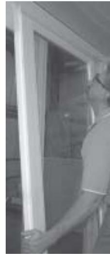
4) Insert the passive panel into the frame with glazing beads towards the inside of the house, by grasping both sides of door panel. Insert top edge into interior frame pocket with the midsection lining up with end of fixed panel and rotate bottom edge over the roller track.
