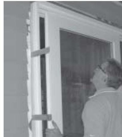
7) Insert the stationary panel, with glazing beads towards the inside of the house & bulb seal end at the bottom, into the frame by lifting it up into the head pocket and then setting it down over the fixed panel setting block. This can be accomplished from either side of the door.
