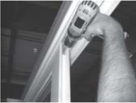
10) Use the (3) #8 x 1/2" PH screws to attach the fixed panel bracket at the head & Panel.
