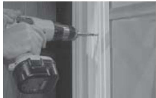
6) Check that frame remains plumb, level, and square using a level and square. Drive #10 x 2 1/2" PH screws into each installation hole, (8) total. 1/2" Screw-hole caps are provided for use when necessary.
