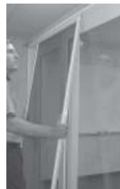
2) Insert the keeper screen into the screen channel on the passive side of the door (on the left from the outside). Insert the screen into the screen channel top end of the screen into the head first. Use a putty knife to push up the bottom rollers when inserting the bottom of the screen into the door.
