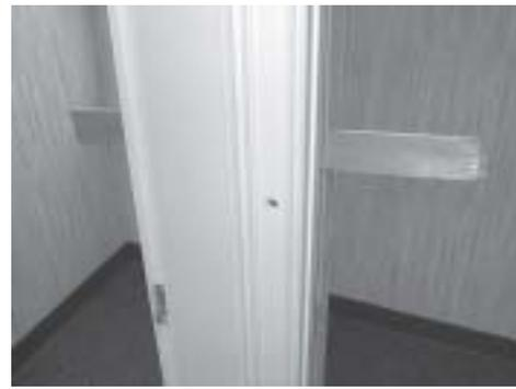
4) Shim jambs and head above each installation hole and head; make sure side jambs do not bow or twist in from the shims. Shims must be placed at the lock jamb behind all locking points. Do not use any shims under sill. The bottom of the frame should set directly on the rough opening floor.
