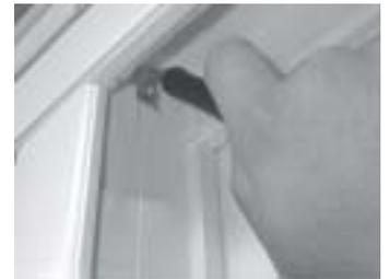
3) Once the Astragal is pushed up against the fixed panel we want to mark the locations for the angle brackets. First place one angle bracket under the sill end of the Astragal where there is a notch in the sill. Mark this location. Second place one angle bracket over the head end of the Astragal in the interior pocket of the head. Mark this location. Note: Both angle brackets will be half covered by astragal when we place astragal on again.
