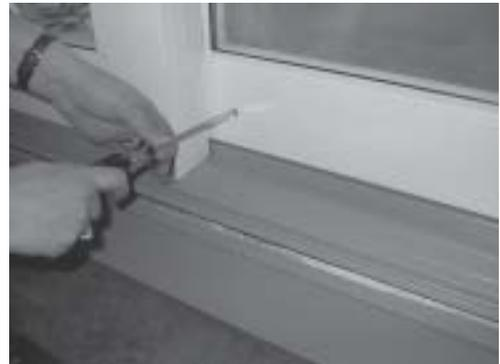
5) Slide panel open and closed to insure ease of operation. If active panel does not slide freely, it may be necessary to re-adjust the roller height.
