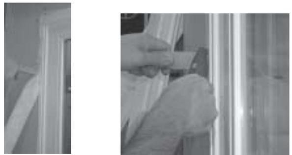
2) Loosely fill remaining gaps at head and jambs with batt type insulation. Do not use expandable foam which may cause frame members to bow.
