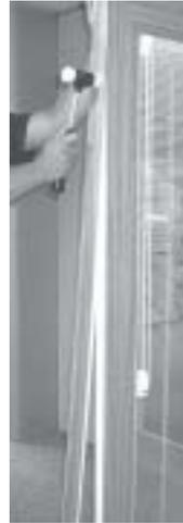
2) While the panel is out, snap in the operating panel interlock (use a rubber mallet if necessary). The interlock must be flush to the bottom of the panel. Start at the bottom and gently tap working your way up the interlock.
