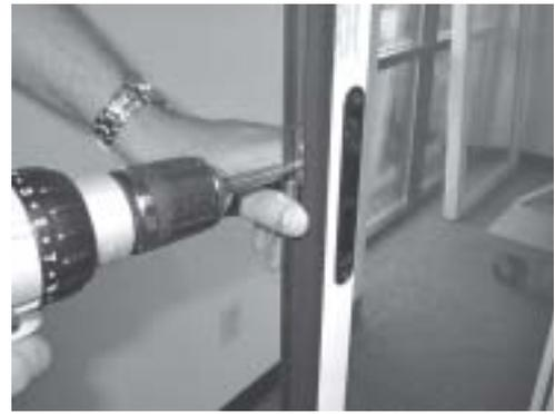
6) Screw in the keeper on the screen mullion on the keeper screen, (use marks that you made to align with lock) use two screws that were attached to the keeper with the screens.
