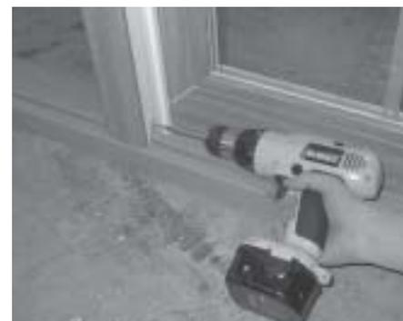
11) Use (2) #8 x 1" self drilling screws to fasten the 1" x 1" angle brackets at the head and sill to the astragal.
