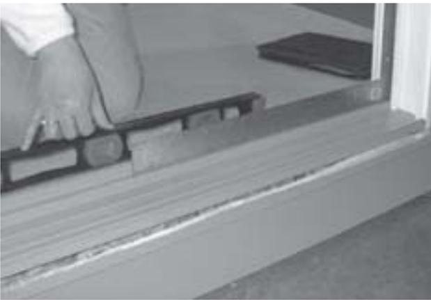
3) Plumb, level, and square frame in rough opening (side to side, front to back and diagonal). Temporarily shim jambs at the extreme corners to keep the frame centered and square. When placing shims, put one inside & one outside to keep the frame from rolling after installation.
