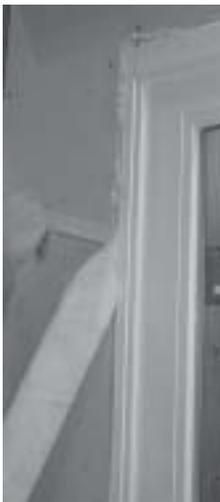
3) Loosely fill remaining gaps at head and jambs with batt type insulation. Do not use expandable foam which may cause frame members to bow.
