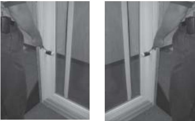
1) Take Jamb Covers and snap into the inner cavity on the jambs (A rubber mallet might be needed). Jamb covers will have one end with a notch in the middle (this end goes towards the sill) and one end with sides notched (this end goes into the head cavity).
