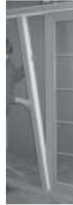
2) Place the Astragal into the frame by first aligning its fabrication at the bottom with the sill. Push the sill end directly against the bottom of the astragal. Do the same with the head end of the astragal.
