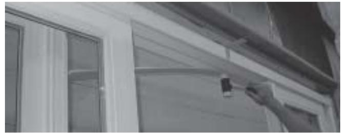
2) Take Head Cover and snap it into the outer cavity on the head (A rubber mallet might be needed). Head Cover will have two 90° ends.
