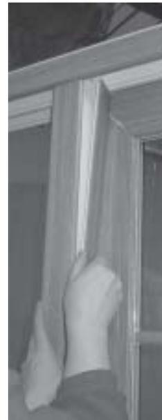
3) Take Interior Astragal Frame Cover and snap into the inner cavity on the Astragal (A rubber mallet might be needed). The Interior Astragal Frame Cover will have one end with a notch in the middle (this end goes towards the sill) and one end with sides notched (this end goes into the head cavity).
