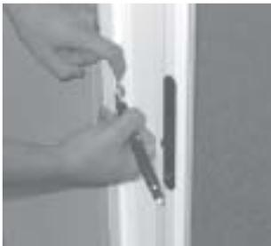
2) Align up the keeper to the lock and mark the keeper on the jamb for keeper location.
