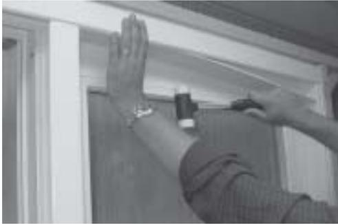
4) Take Head Cover and snap one into the outer cavity on the head & one into inner cavity on the head next to the astragal. (A rubber mallet might be needed). Head Covers will have two 90° ends.
