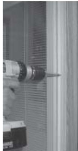
3) With the exterior of the panel facing you, locate a vertical groove next to the interior weather strip on the interlock. Use (5) #8 x 1" PH self drilling screws to fasten through the interlock into the face of the panel. Evenly space the screws down the full length of the interlock, use the same locations as the fixed panel interlock.
