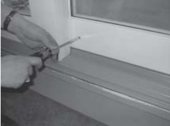
5) Slide panel open and closed to insure ease of operation. If active panel does not slide freely, it may be necessary to re-adjust the roller height. Take the weight off the panels for adjusting the rollers using a shim. To extend the rollers turn clockwise and to retract the rollers, thurn counter clockwise.
