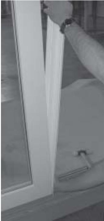
12) Snap in the fixed panel interlock (use a rubber mallet if necessary). The interlock must be flush to the bottom of the panel. Start at the bottom and gently tap working your way up the interlock. If necessary, trim bulb seal even with bottom of panel on the interlock.
