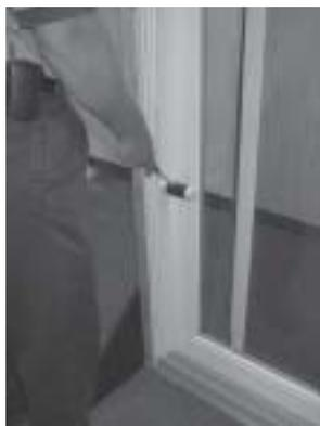
2) Take Jamb Covers and snap one into the inner cavity on the jamb & one into the outer cavity on opposite jamb (A rubber mallet might be needed).
