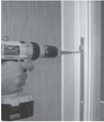
2) Once the keeper(s) are in position, replace the short factory installed screws with (8) #10 x 3" Flat Head screws. These long screws will insure that the keepers stay in place.
