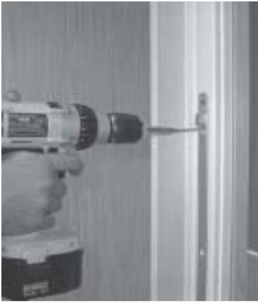
1) The keeper(s) are installed at the factory. Test the keeper locations by operating the lock. Make sure the active panel is fully engaged while testing the keeper position(s). If needed you can move the keeper by backing out screws and repositioning keeper.
