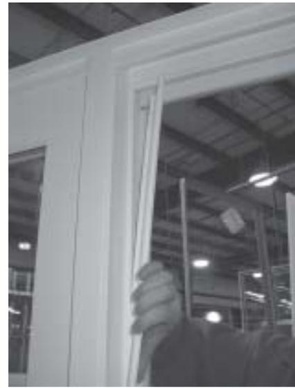
2) Take Exterior Astragal Frame Cover and snap into the outer cavity on the Astragal (A rubber mallet might be needed). The Exterior Astragal Frame Cover will have one end with a 3° angle cut (this end goes towards the sill) and one end with the sides notched (this end goes into the head cavity).
