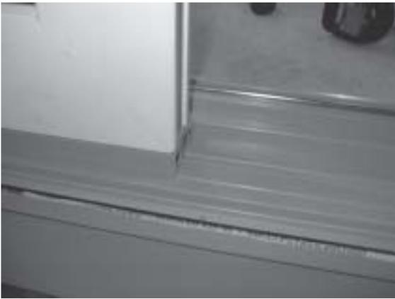
8) Slide the panel along the setting block into the jamb pocket. Check to make sure the panel is installed all the way back into the jamb pocket. Use a rubber mallet to tap the panel in place and align with the end of the setting block.
