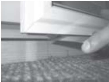
1) Insert the screen into the screen channel top end of the screen into the head first. Use a putty knife to push up the bottom rollers when inserting the bottom of the screen into the door.
