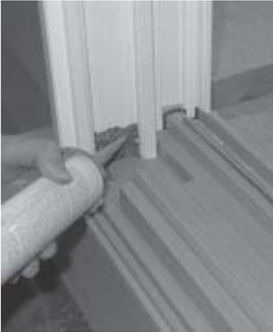
2) Place a back bead of silicone in the exterior sash pocket of the fixed jamb. This silicone should be placed around the sill joint and to a height equal to the fixed panel setting block that will be installed in the next step.
