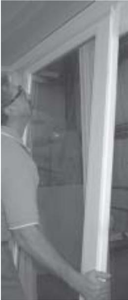
4) Insert the active panel into the frame with glazing beads towards the inside of the house, by grasping both sides of door panel. Insert top edge into interior frame pocket with the midsection lining up with end of fixed panel and rotate bottom edge over the roller track.
